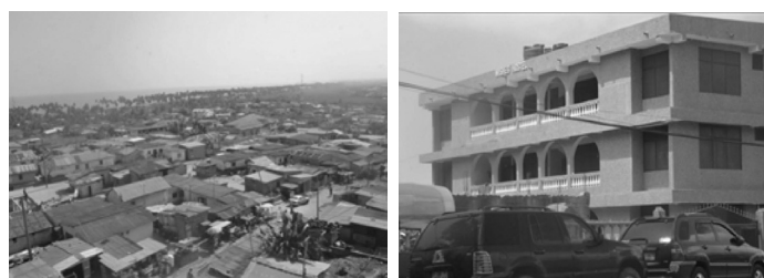
Unsafe and safe areas
